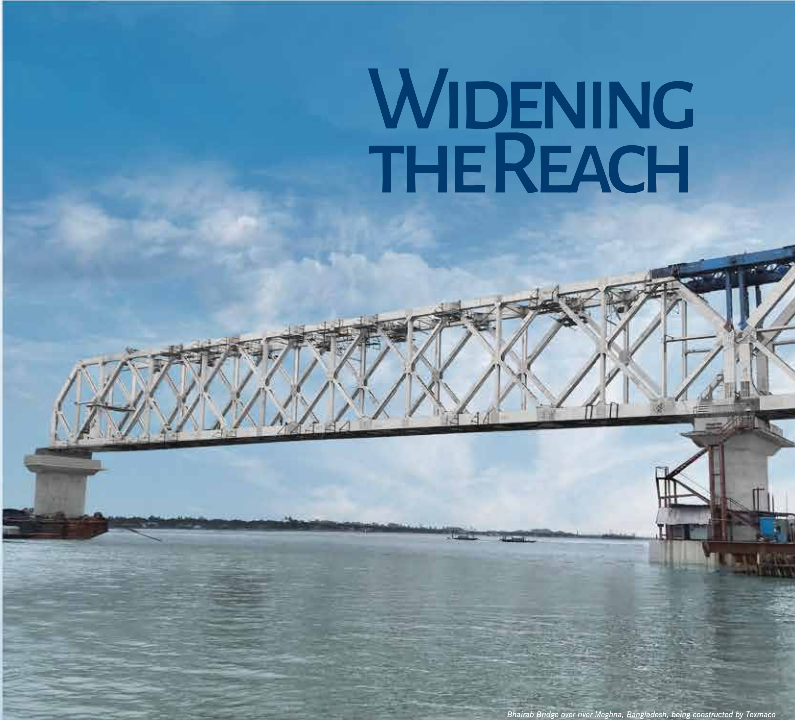
Bhairab Bridge over river Meghna, Bangladesh, being constructed by Texmaco
