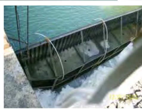
Closer view of one of the new gates in operation
