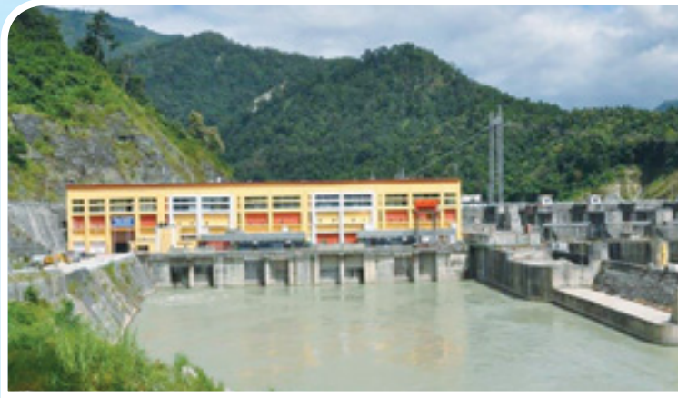
Teesta Low Dam (Stage III) 130 MW Hydro Electric Project in West Bengal Conception to Commission by Texmaco
