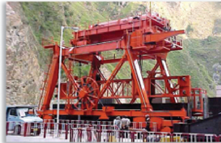
▲ 230T Spillway Gantry Crane Chamera-II - HP
