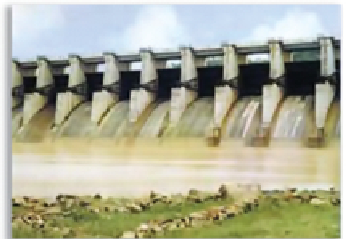
Rope Drum Hoist Operated Spillway Gates. 99 MW OBRA DAM, Uttar Pradesh
