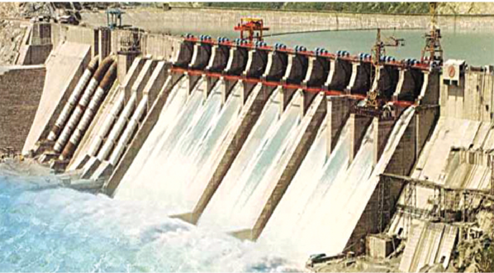
Rope Drum Hoist Operated Spillway Gates. 345 MW Salal H.E. Project, J & K
