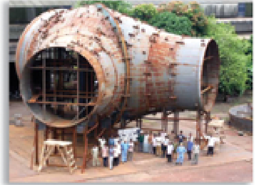
3-Piece Junction Purulia Pumped Storage Project West Bengal
