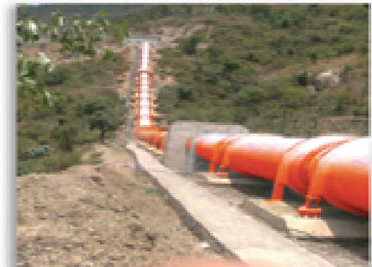
Surface Penstock Sewa II, H.E. Project, J & K.
