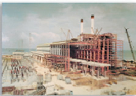
Steelwork and Cladding Tuanku Ja'far Thermal Power Station, Malaysia
