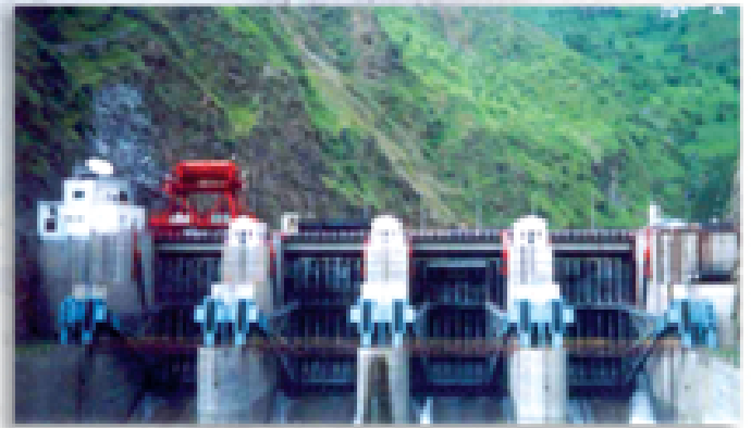
Hydraulic Hoist Operated Spillway Gates. The largest in India and second largest in the World. 300 MW Chamera-II H.E. Project, Himachal Pradesh
