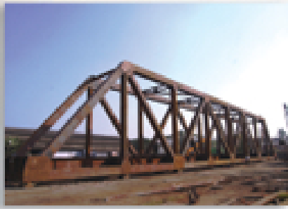
Rail Link Triangulated Bridge Dhamra, Bhadrak, Orissa
