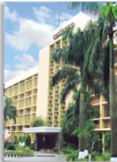
Administrative Building Birla House
