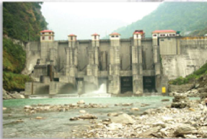
Hydraulic Hoist Operated High Head Spillway Gates. 510 MW Teesta-V H.E. Project, Sikkim
