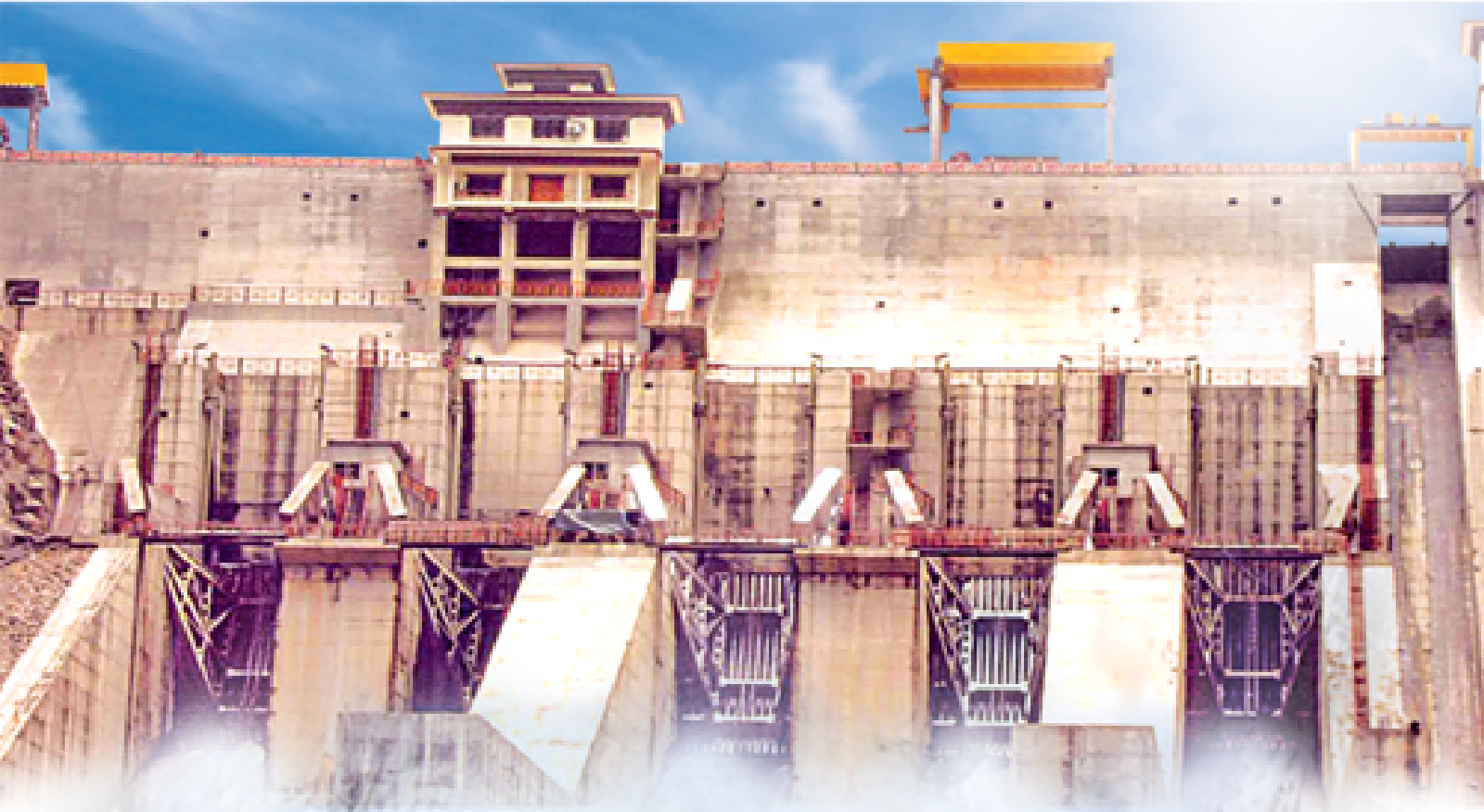
Hydraulic Hoist Operated High Head Spillway Gates. 1020 MW Tala H.E. Project, Bhutan
